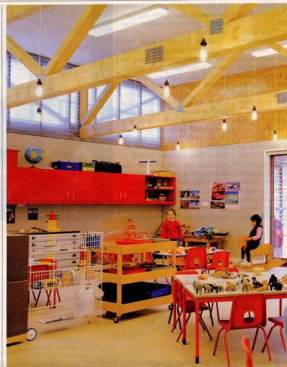
Left: Nursery space, surmounted by 1.2m-deep timber trusses. Right: Stair between the community café and the facilities on the upper ground floor.
